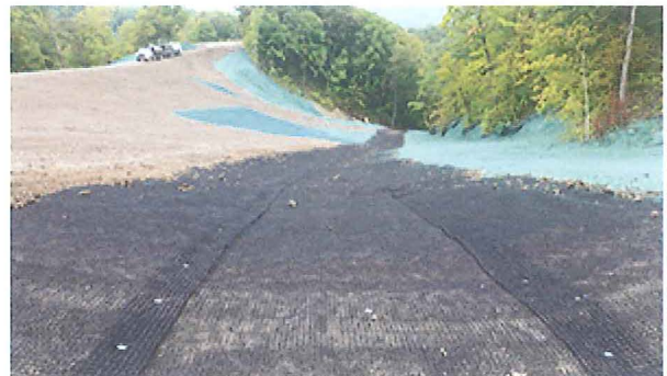
Credit: BARR ENGINEERING TRMs and Flexterra hold the slope in place.
